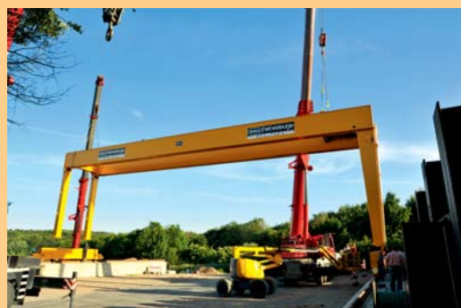
Fitting the crane structural to the end carriages
