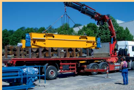
Delivery of the single components
