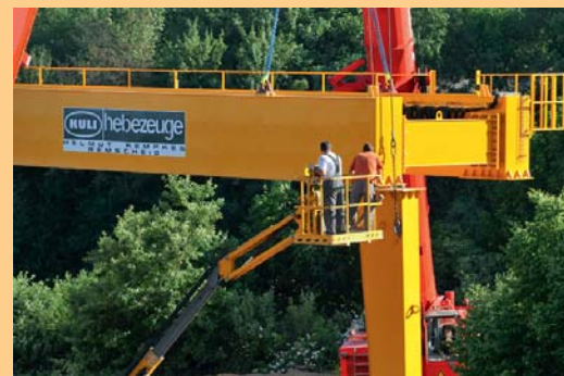
Assembly of the fixed column
