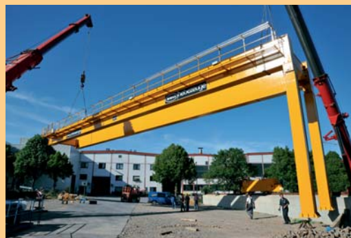
Erection of the crane without fixed column
