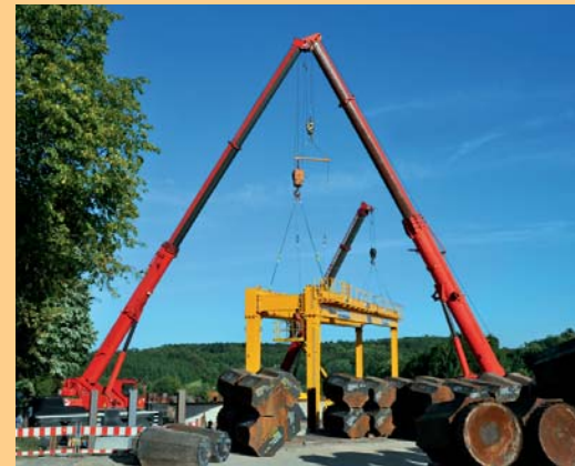
Assembly by truck mounted cranes
